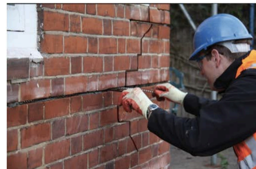
Figure 4 - Typical image of Helifix crack stitch method where mortar joints are raked out, helical bars inserted and grouted/resin injected in order to reinforce the wall panel
