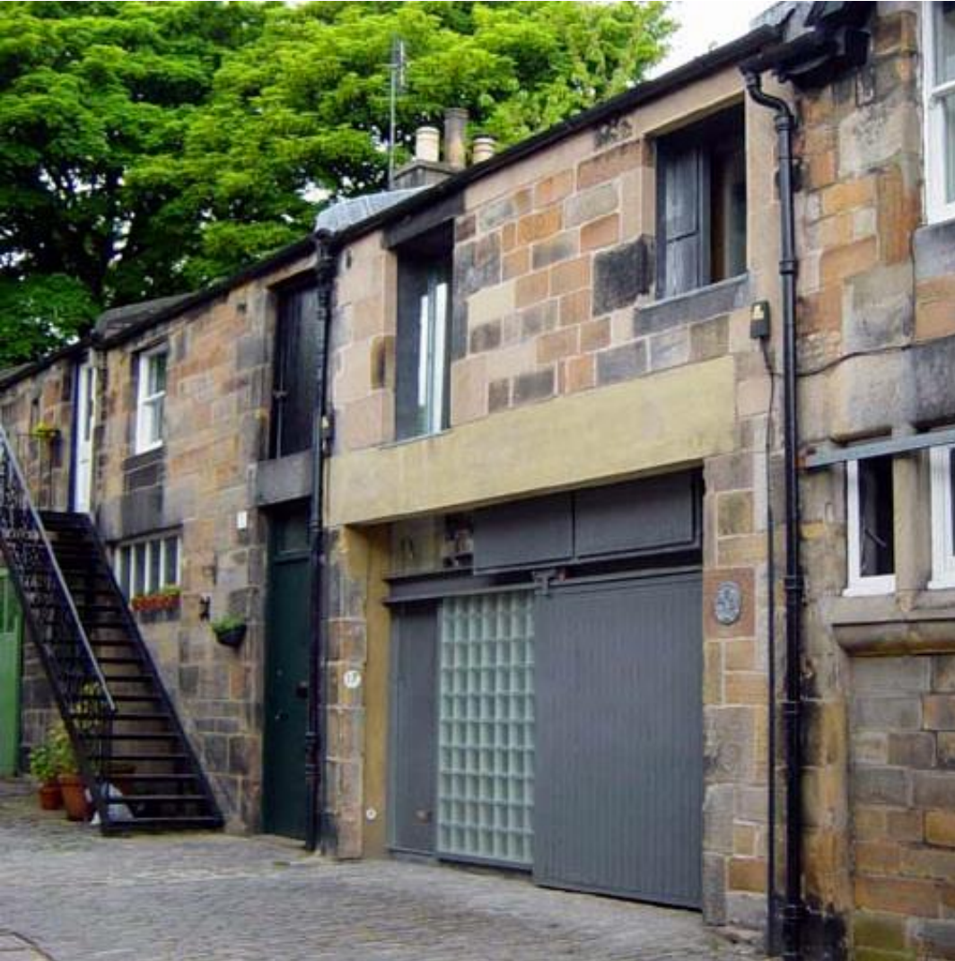
Stables converted into a house in Edinburgh – Richard Murphy Architects
