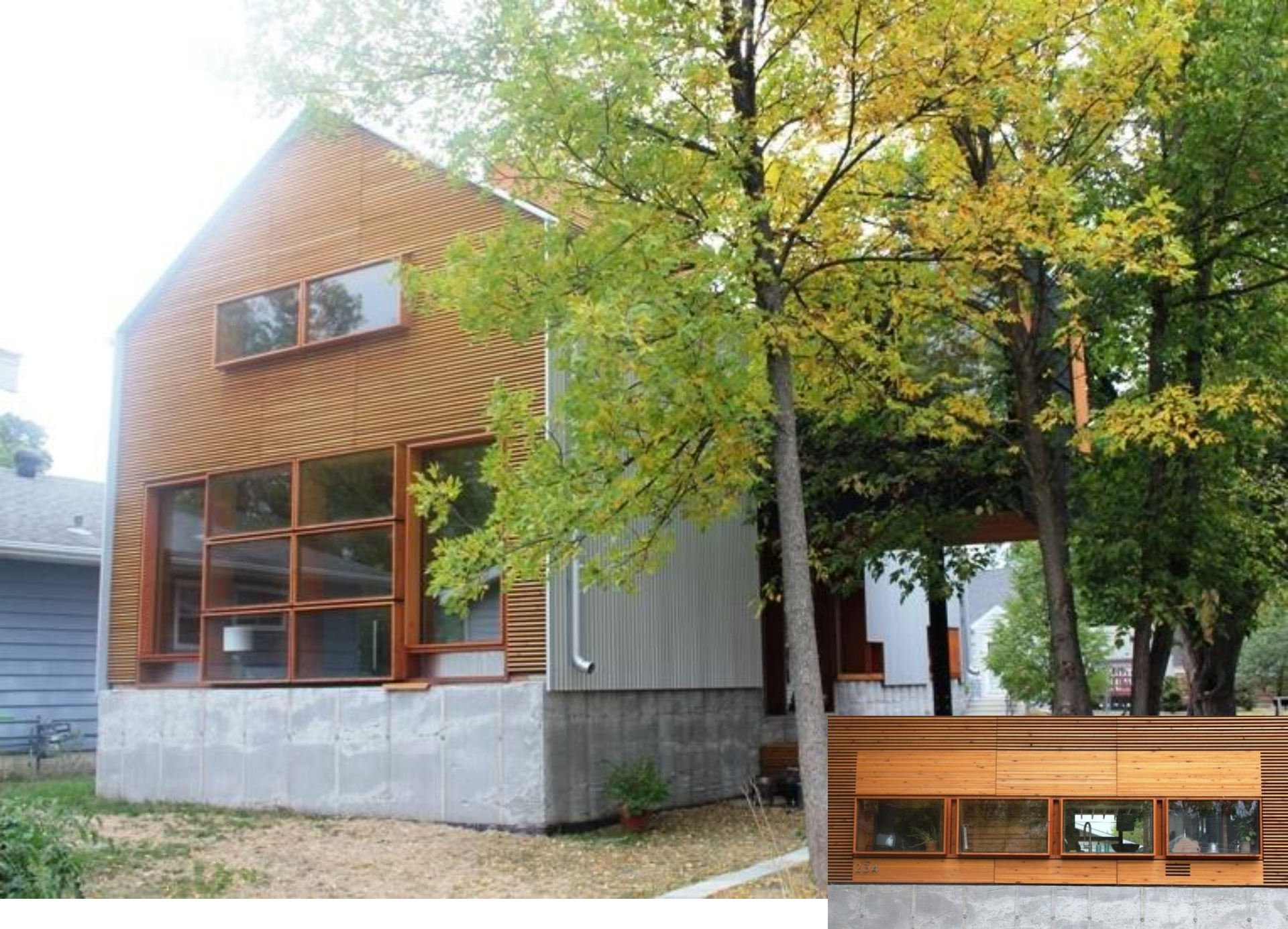
Cloud House designed to make use of reclaimed of glazed units, Regin Schwaen , Professor North Dakota State University
