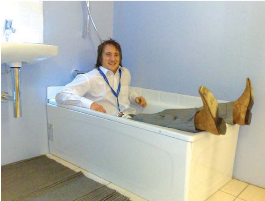
Figure 2. A 1300mm long, 110 litre bath installed for CSH compliance.
