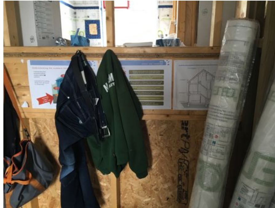
Construction approach was not clear to people building it
