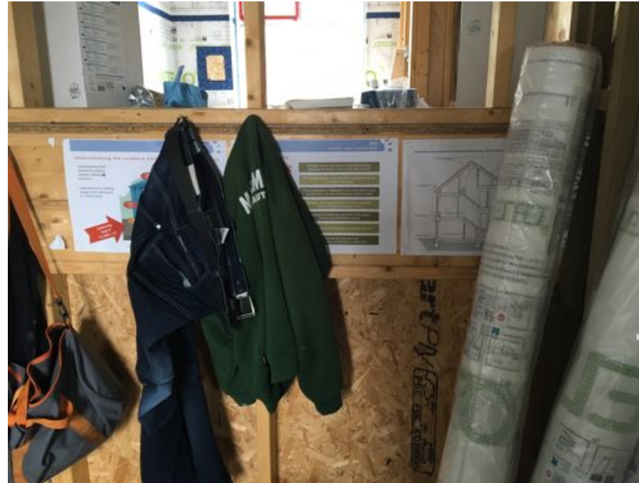
Construction approach was not clear to people building it
