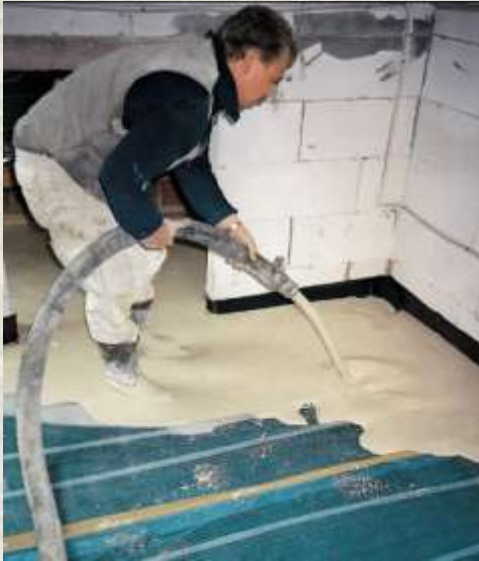
Fig.: Screed installation
