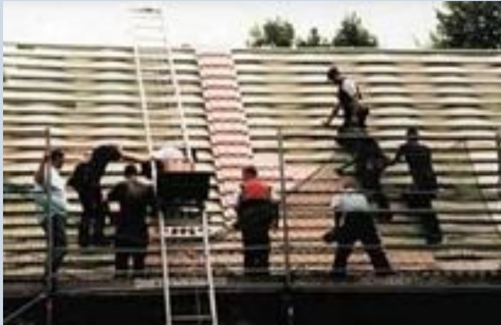
Fig.: A new construction of a roof
