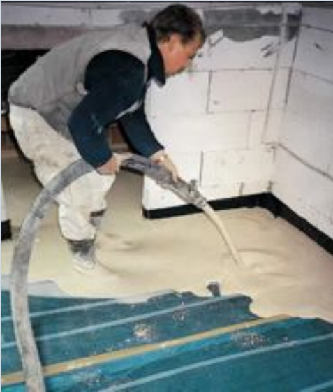
Fig.: Screed installation
