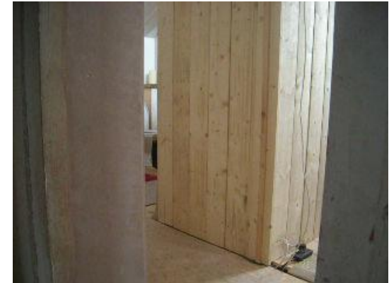
Video clip – hot water & secondary heating system
