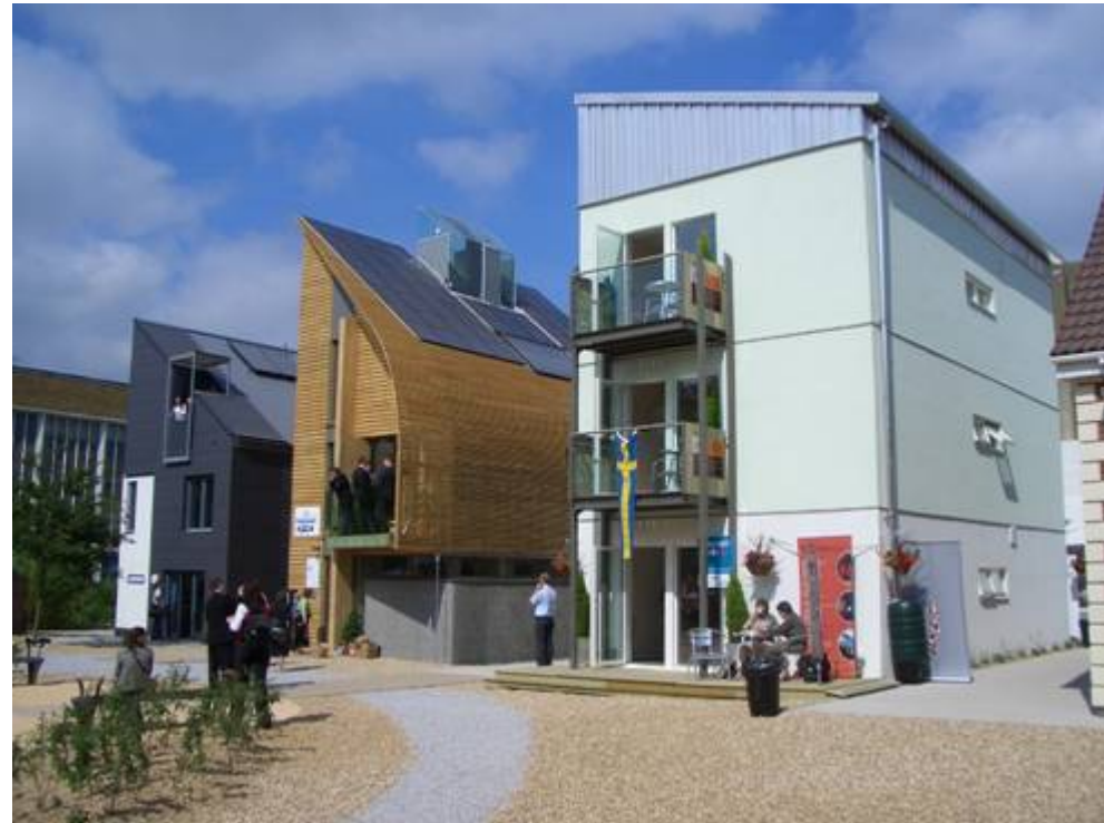
3 prototype houses at BRE Innovation Park, UK
