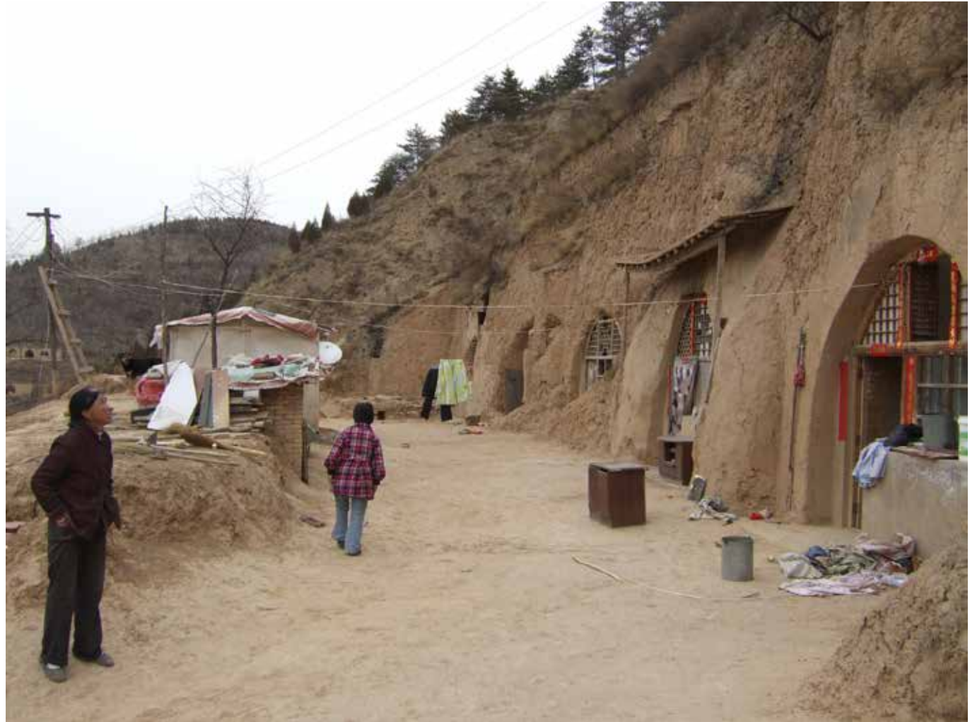
New Generation Cave Dwellings Zaoyuan Village, Yan'an, Shaanxi, China Case Study Visited March 2011
