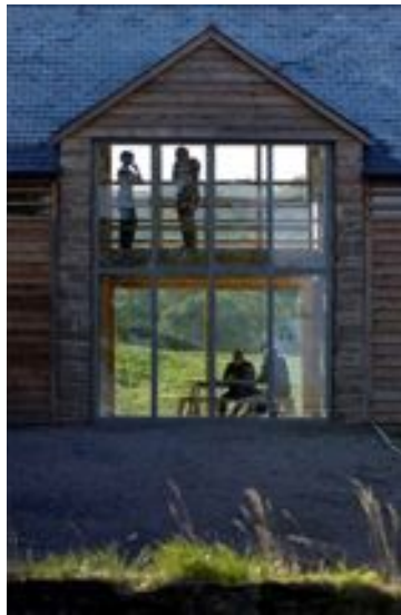
West Office - Barn Ecological refurb
