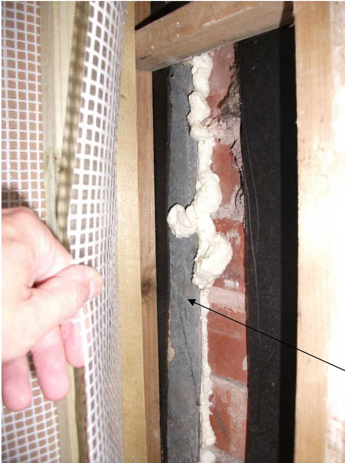
Original metal cavity closer sealed with expanding foam to make air tight.
