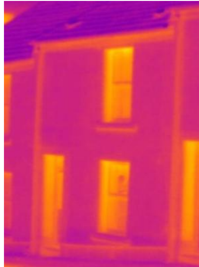
Assessing the execution of retrofitted external wall insulation for pre-1919 dwellings in Swansea (UK); Joanne Hopper et al 2011
