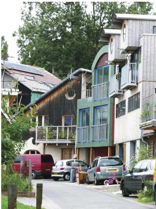
Another view from the Ashley Vale site visit.
