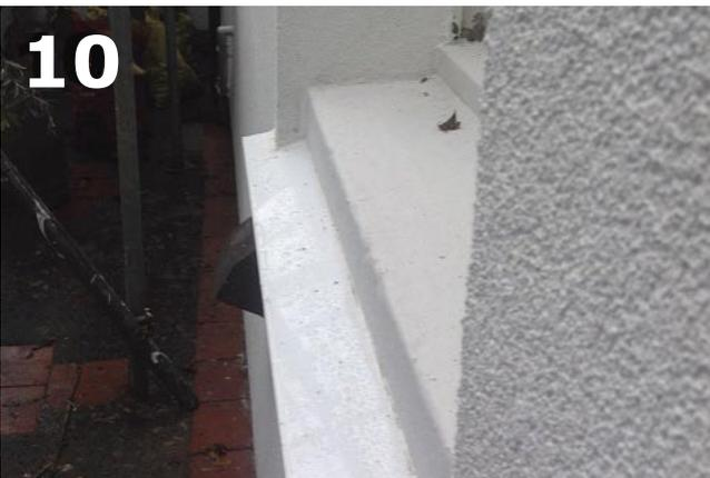
However, at Somerset Road a bespoke insulated over-sill was proposed, being preferable as the main intention was to eliminate, or at the least diminish, the thermal bridging effect of the existing concrete cills.
