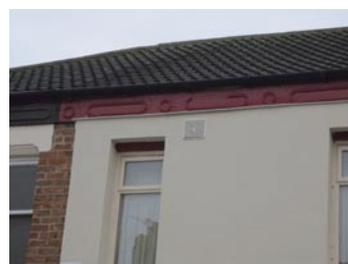
Leaving the decorative band at the top of this wall exposed has created a large thermal bridge, and may increase the risk of rain penetration. Courtesy NDM Heath Ltd
