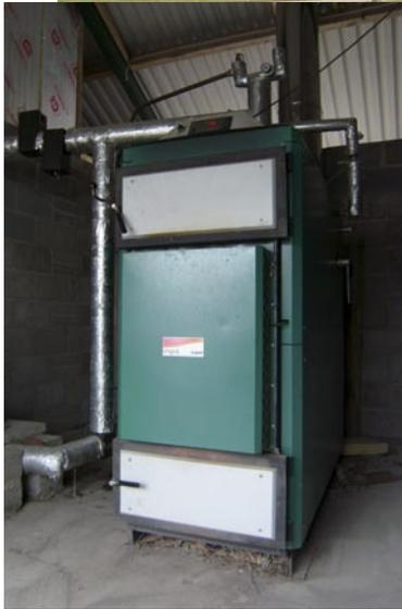
capable of burning logs, with a moisture content of 15-20%, up to 100cm in length. The solution works at 91% efficiency and can burn for up to 12 hours continuously. This high efficiency means that, during the summer months, a single weekly load will ensure enough hot water is provided to every building on site.
