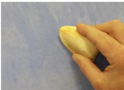
Tadelakt is a polished plaster originating from the Mediterranean region of Morocco and means 'to rub' or 'knead' in Arabic. The application of Tadelakt had a practical purpose in a hot, arid climate and records indicate that nomads used it to seal reservoirs for
