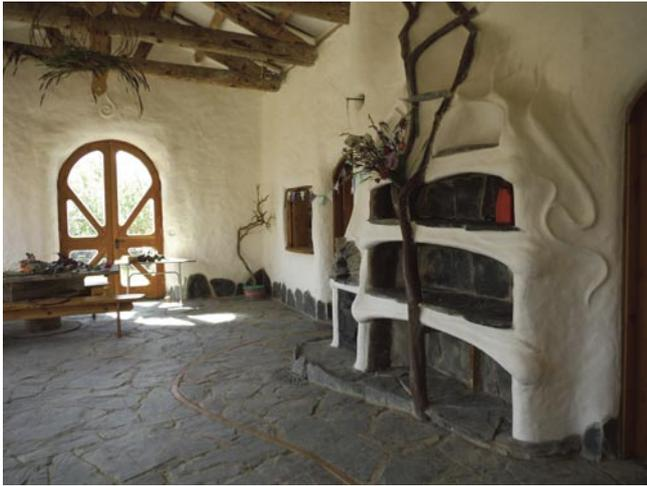
Left: the interior of the hub, with the typical contoured effect created by lime rendered straw bale walls.
