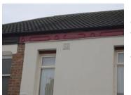
Leaving the decorative band at the top of this wall exposed has created a large thermal bridge, and may increase the risk of rain penetration. Courtesy NDM Heath Ltd
