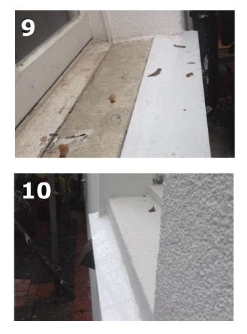
However, at Somerset Road a bespoke insulated over-sill was proposed, being preferable as the main intention was to eliminate, or at the least diminish, the thermal bridging effect of the existing concrete cills.
