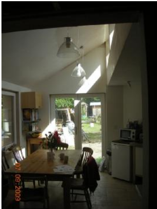
South facing vertical windows in extension and refurbished roof –
