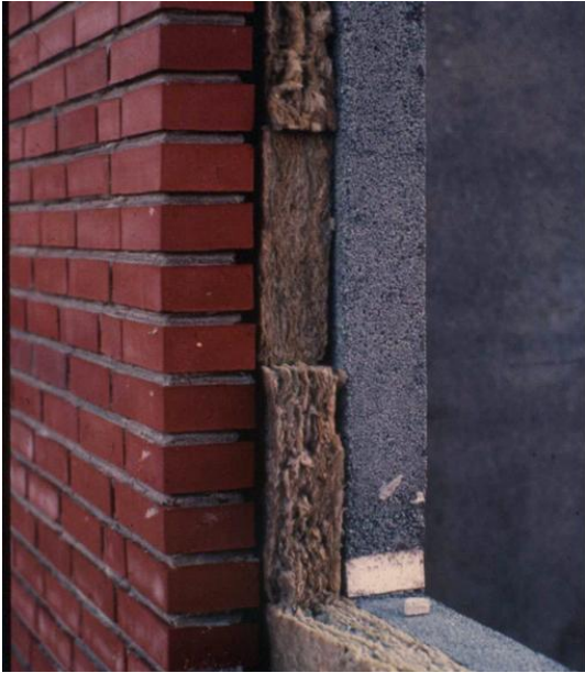
Figure 24. New cavity wall in Denmark in 1977.
