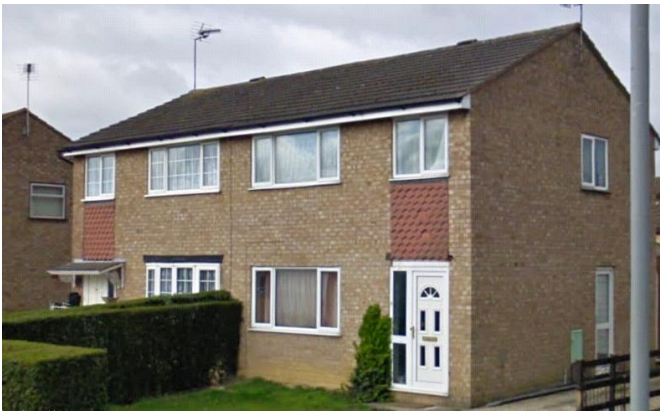
Figure 38. Cavity-walled semi-detached houses.
