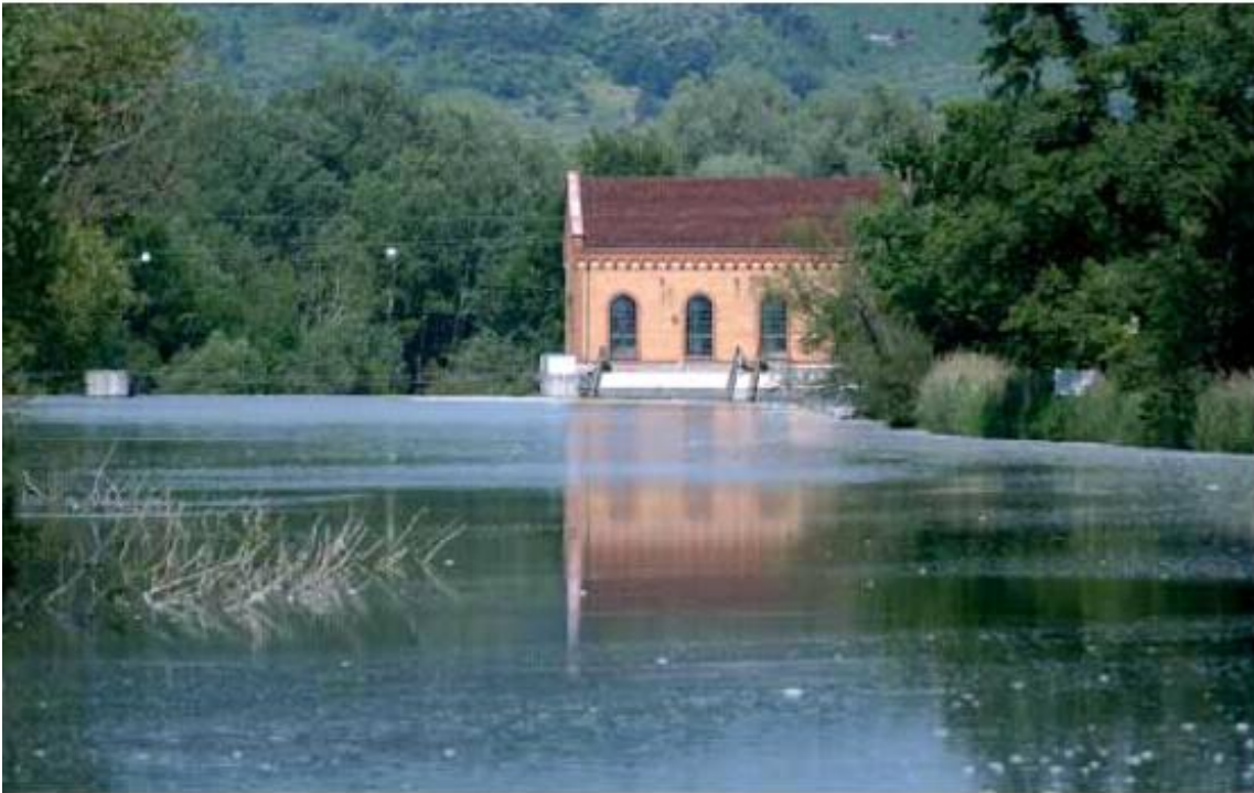
Figure 18. Hydroelectric power plant on the River Neckar at Kiebingen, Germany. 204 Courtesy: Energie Baden-Württemberg AG.
