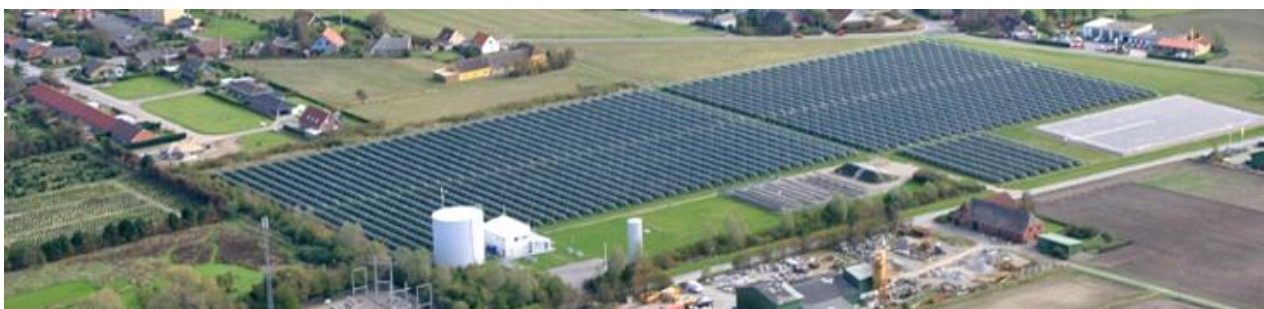
Figure 15. Solar collectors of the Marstal DH system.
