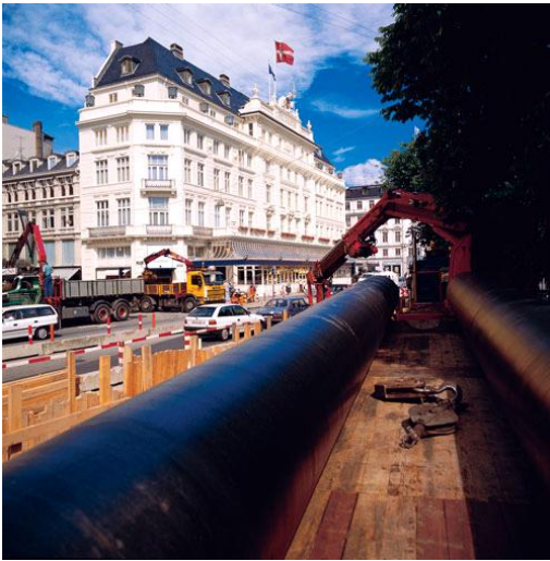
Figure 33. Large heat main being laid in Copenhagen. 373
