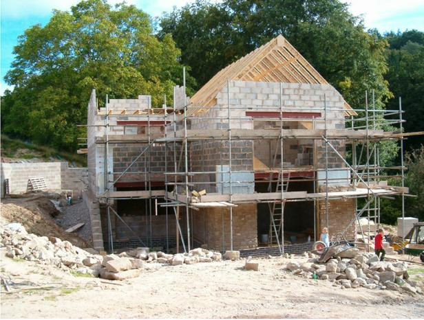
(2) Wall type 2: externally-insulated and rendered wall. 13mm dense plaster, 100mm dense concrete block, 200mm blown cellulose fibre between 'TJI' I beams on 600mm centres, 9 mm 'Panelvent' sheathing, breather membrane, 50mm cavity, 20mm render on stainless steel lath.
