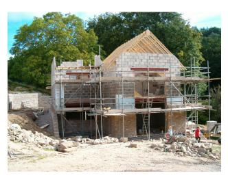
(2) Wall type 2: externally-insulated and rendered wall. 13mm dense plaster, 100mm dense concrete block, 200mm blown cellulose fibre between 'TJI' I beams on 600mm centres, 9 mm 'Panelvent' sheathing, breather membrane, 50mm cavity, 20mm render on stainless steel lath.
