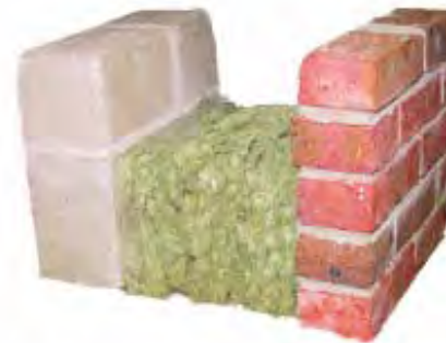
thermal mass and insulation at BedZED
