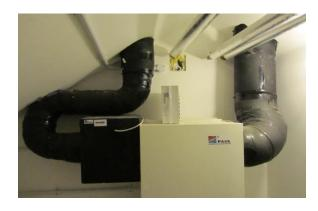
Fig 2. Passivhaus design specifies vapour retardant insulation, to prevent condensation forming inside or outside the ventilation ducts
