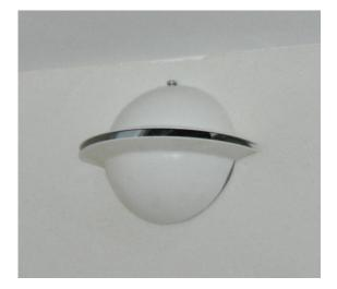
Fig 3. Ventilation outlet in a Passivhaus – the air moves over the ceiling before gently mixing with the air in the room
