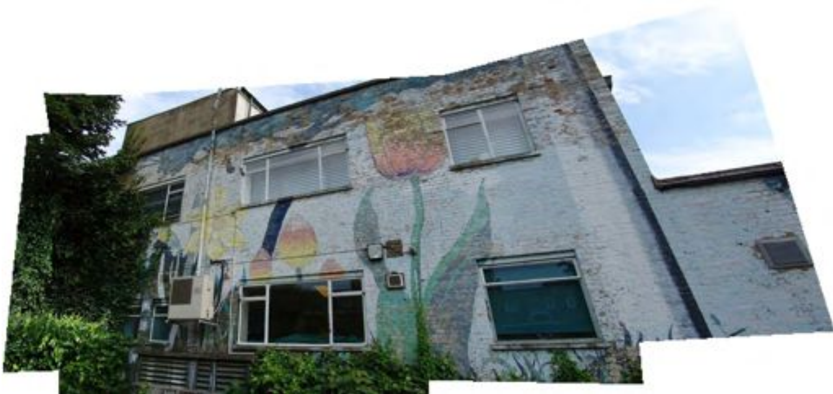
South elevation before refurbishment
