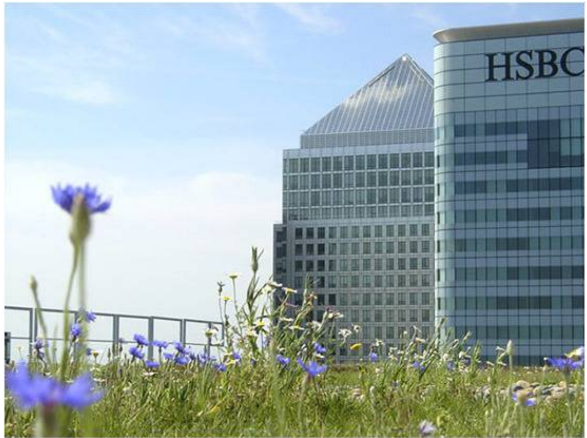
Roof of Barclays Tower, Canary Wharf – at the time the highest green roof in Europe
