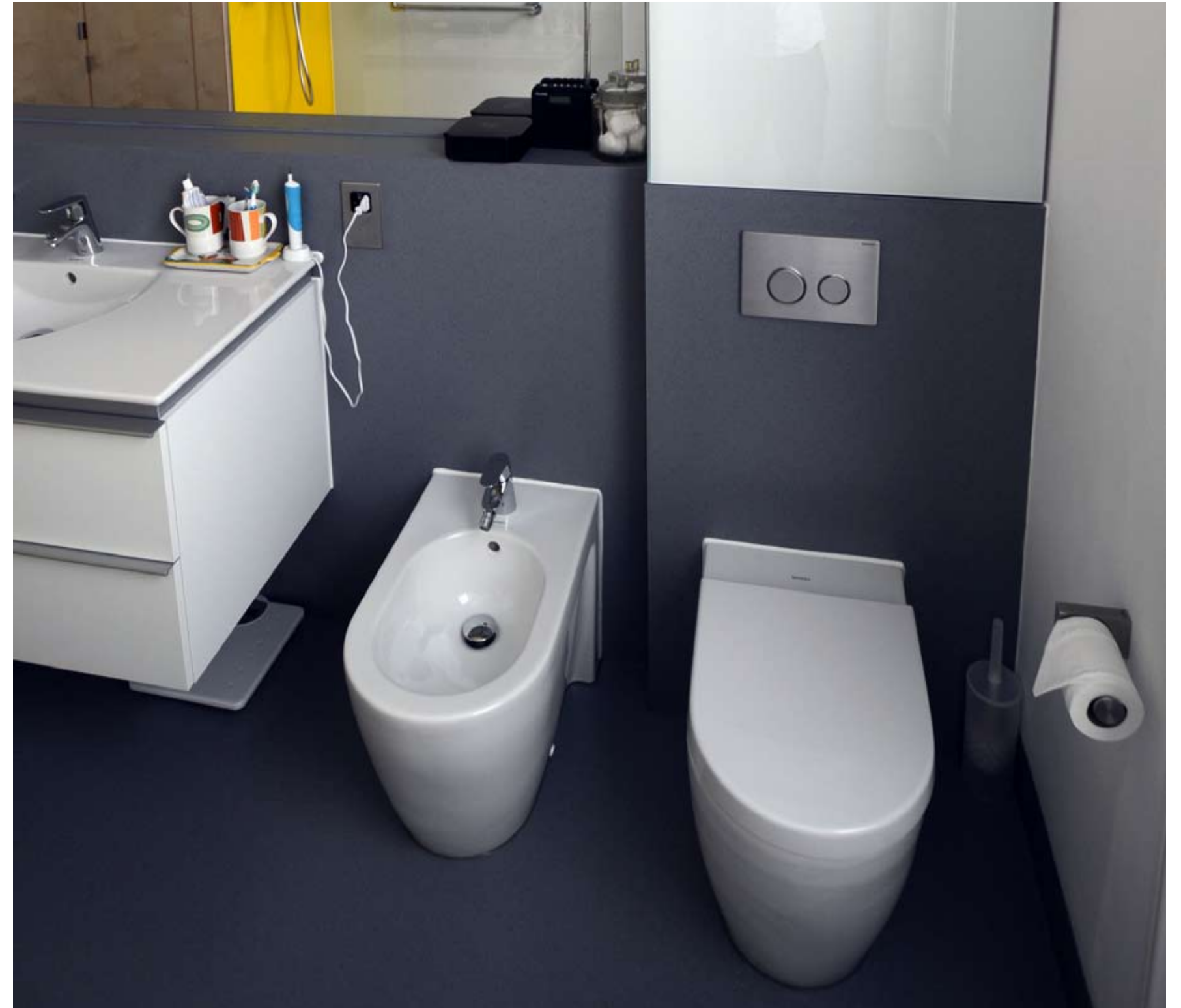
1st floor shower room
