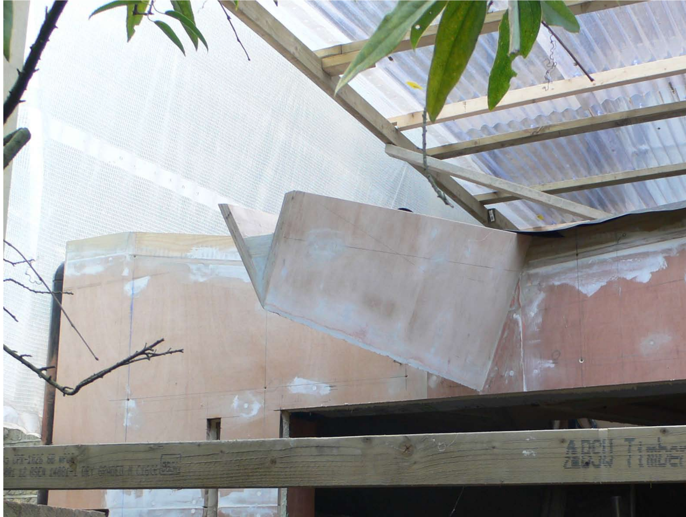
rain garden spout under construction
